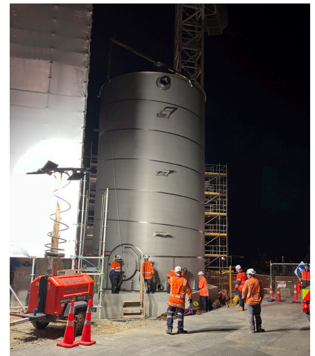
The first of five new spiral-welded tanks was installed on Thursday night.
